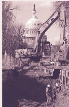
Figure E5.5a (Photo courtesy of Architect of the Capitol.)
