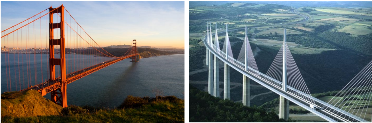
Figure 4.1 Suspension bridge (Golden Gate Bridge) and cable-stayed bridge (Millau Viaduct, France).
