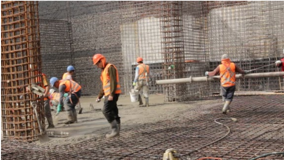
Figure 15-2 Casting concrete in a reinforced concrete building.
