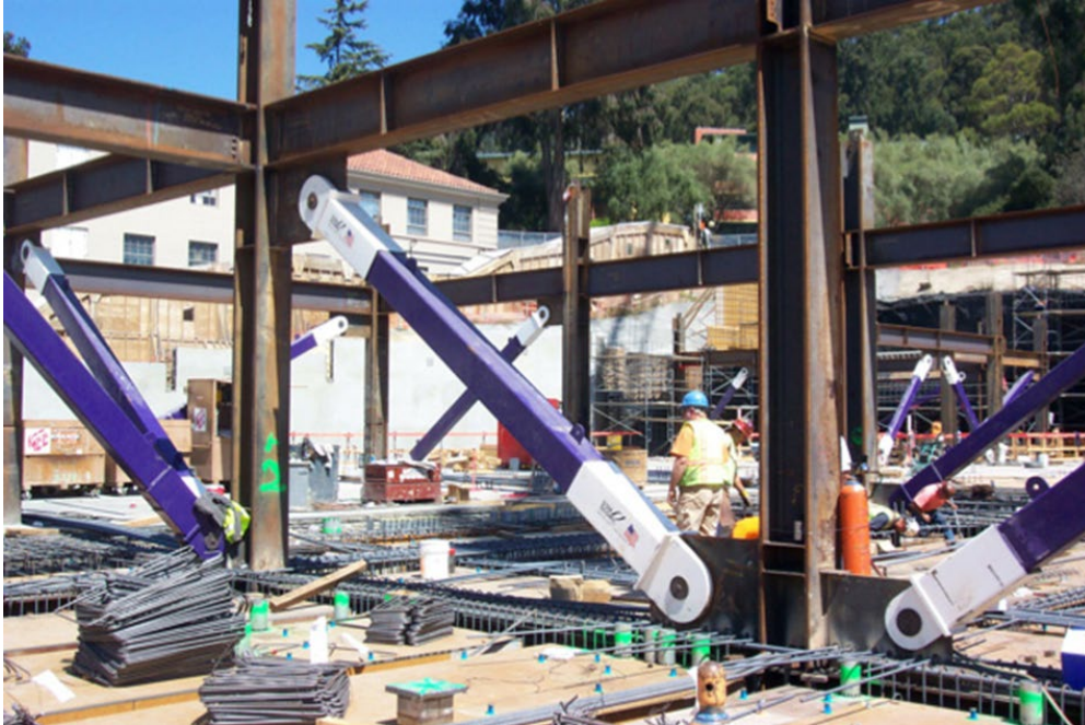
Figure 11.18 Buckling-restrained braced frame in Stanley Hall, UC Berkeley.
