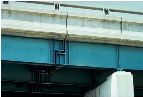
(a) Bridge structure
