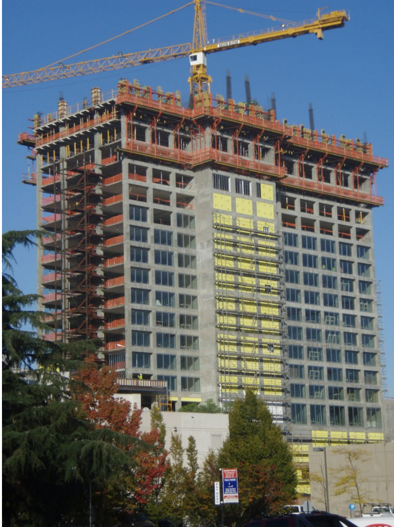
Figure 11.16 Reinforced concrete moment-resisting frame under construction (Cary Kopczynski & Company, Seattle).
