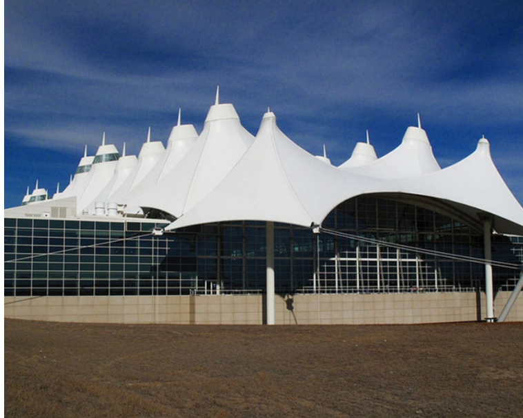
Figure 4.2 Tensile membrane structure (Denver International Airport).
