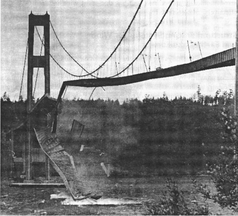
Photo 2.1: Failure of the Tacoma Narrows Bridge showing the first section of the roadway as it crashes into Puget Sound. The breakup of the narrow, flexible bridge was produced by large oscillation induced by the wind.
