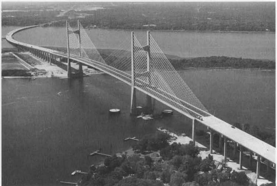
FIGURE 1.8 Napoleon Bonaparte Broward Bridge, with a 1300 ft center span at Dame Point, Jacksonville, Florida. (HNTB Corporation, Kansas City, Missouri.)
