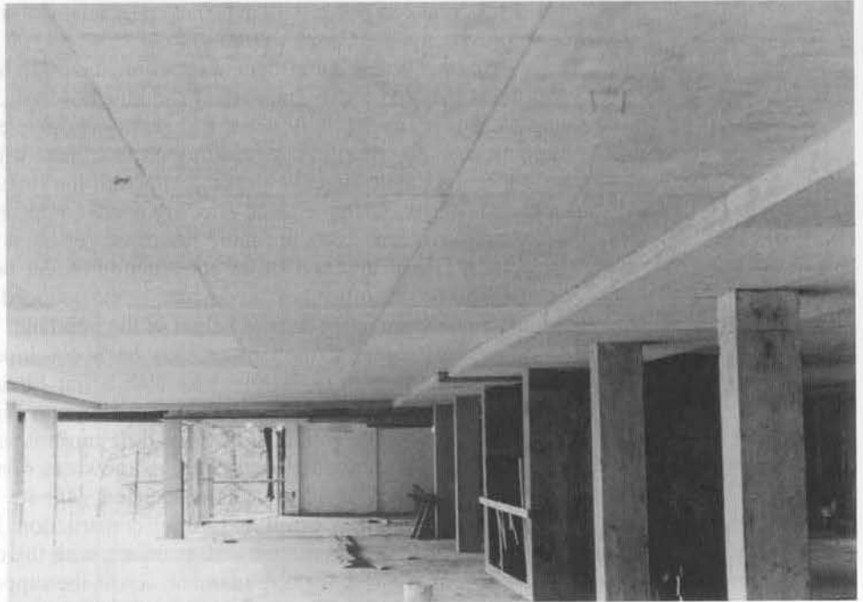
(a) Interior slab band
