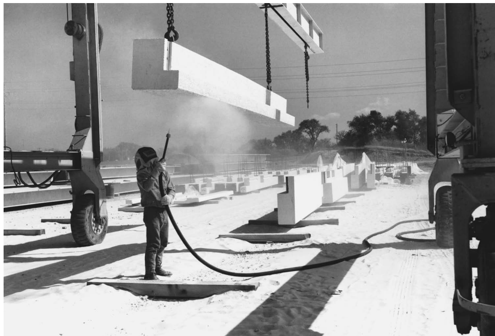
FIGURE 19.19 Sand-blasted architectural finish applied to a precast L beam. (Photograph by Charles W. Dolan.)
