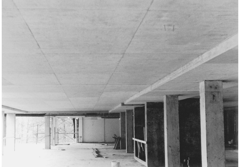
(a) Interior slab band
