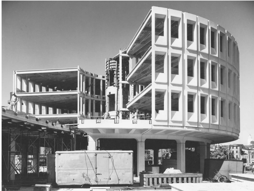
FIGURE 19.22 All precast administration building. (Courtesy of Portland Cement Association.)
