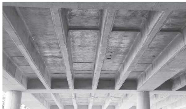
(b) Section X-X joist floor system
