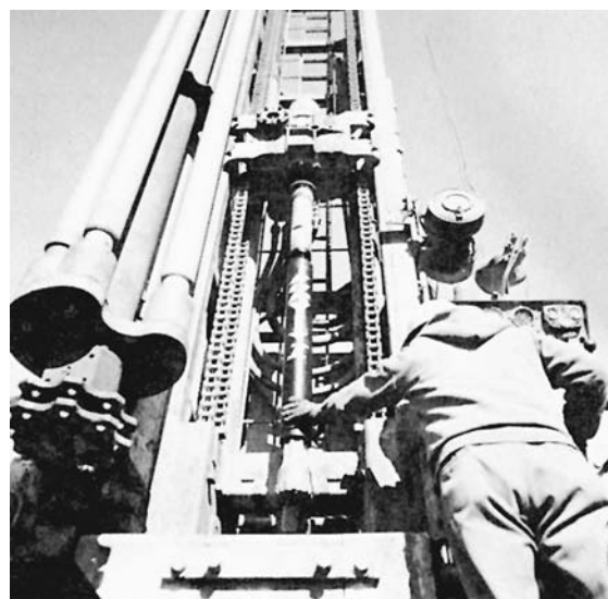
FIGURE 8. Downhole drill mounted on a rotary drill. (Courtesy of Ingersoll-Rand Company)
