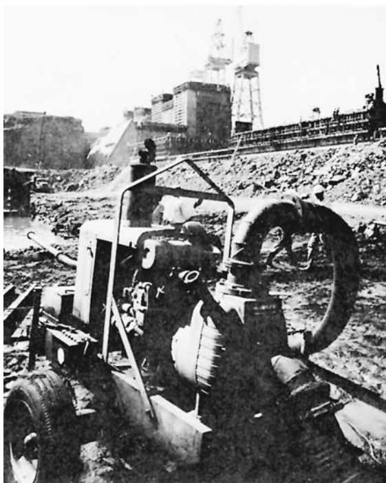
FIGURE 7. Self-priming centrifugal pump at dam construction site. (Reproduced with permission from the Association of Equipment Manufacturers)
