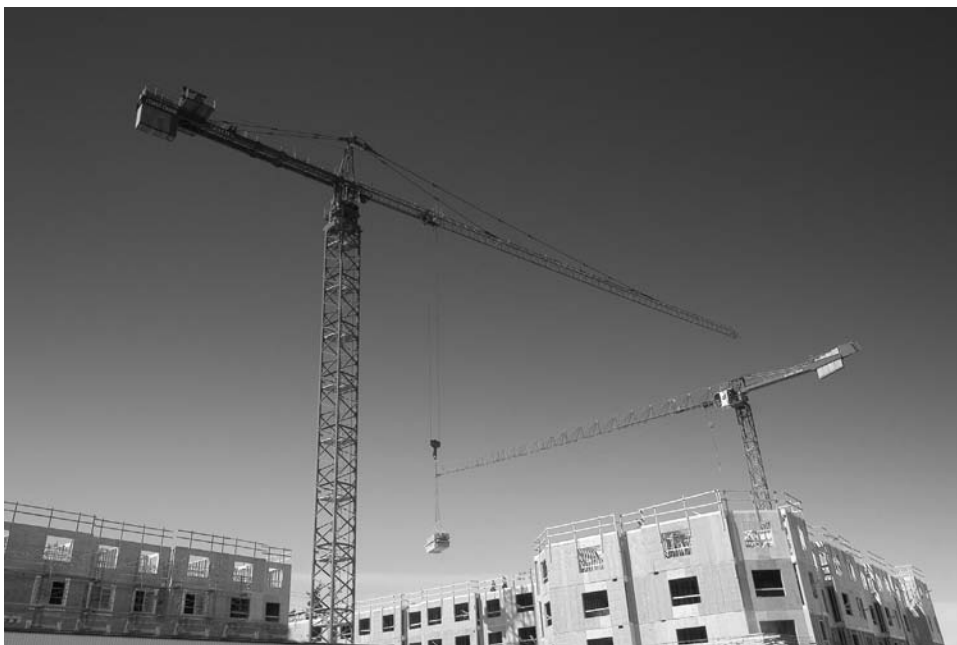
FIGURE 28. Tower crane on a building site. (Courtesy of Manitowoc)
