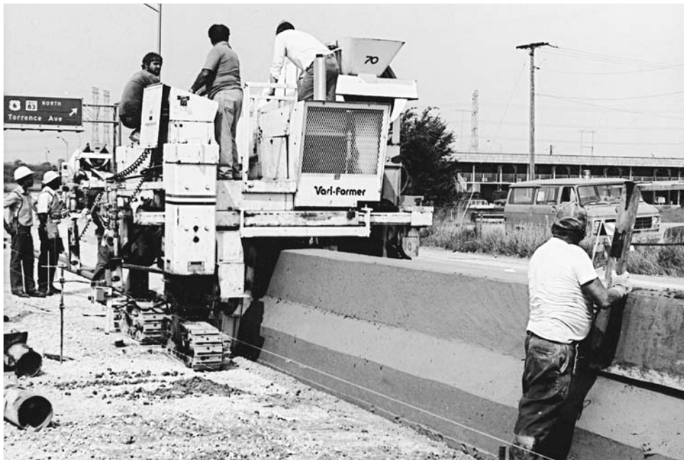
FIGURE 3. Slipform paver placing median barrier. (Reprinted Courtesy of Caterpillar Inc.)
