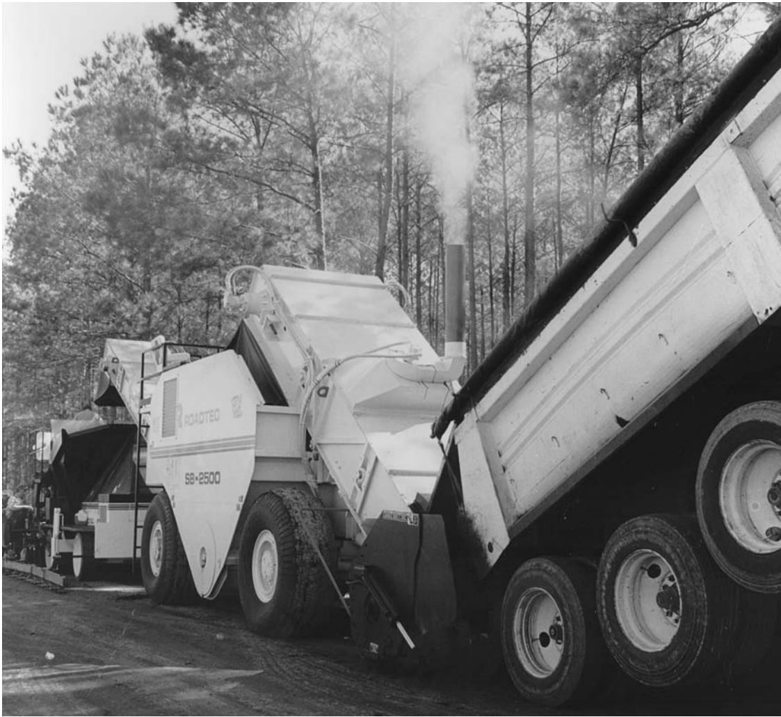
FIGURE 6. Material transfer vehicle feeding an asphalt paver. (Courtesy of Roadtec, Inc.)
