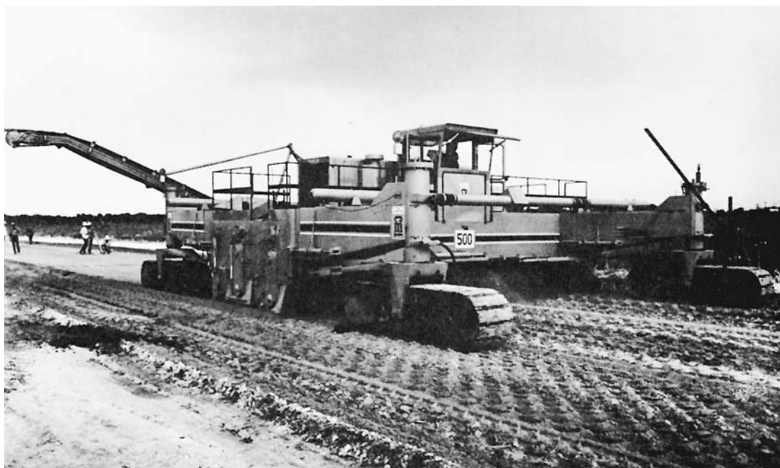
FIGURE 17. Large-grade trimmer/reclaimer/paver. (Courtesy of Terex Roadbuilding)
