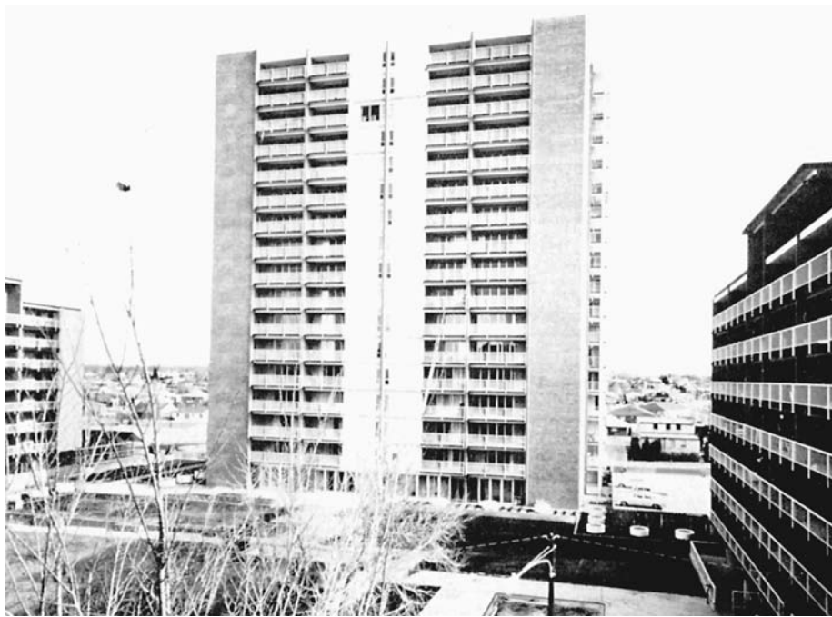
FIGURE 10. Seventeen-story building constructed with reinforced brick masonry bearing walls. (Courtesy of Brick Industry Association)
