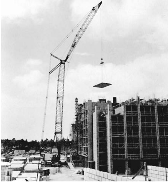
FIGURE 26. Repositioning flying form. (Courtesy of CMI Terex Corporation)
