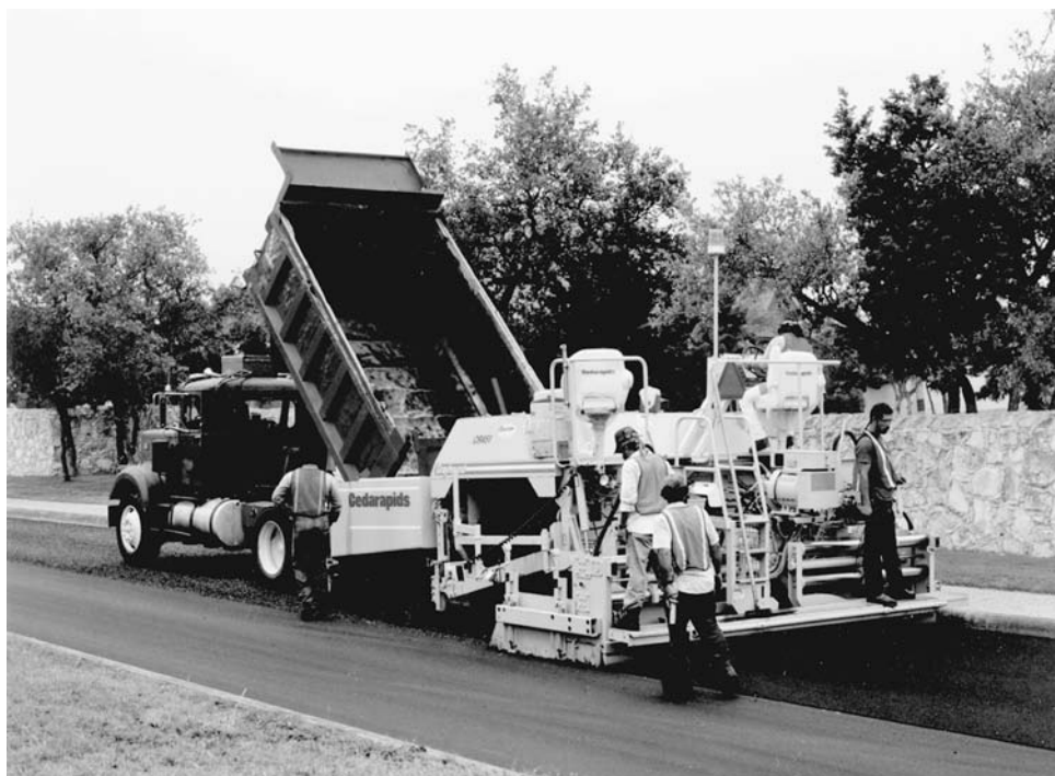
FIGURE 5. Asphalt paving machine in operation. (Courtesy of Cedarapids, Inc.)
