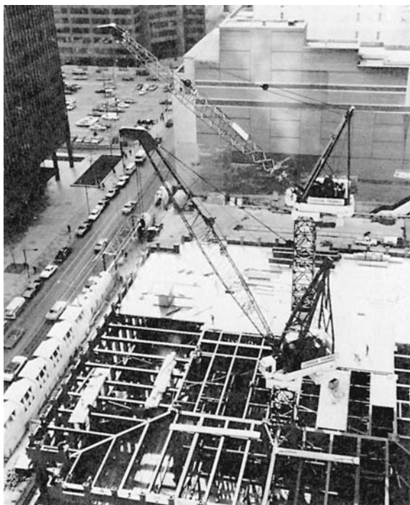
FIGURE 9. Tower crane erecting steel. (Courtesy of FMC Corporation)
