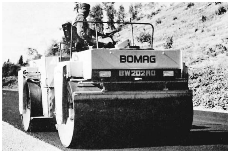
FIGURE 8. Rolling an asphalt pavement with vibratory roller. (Courtesy of BOMAG [USA])
