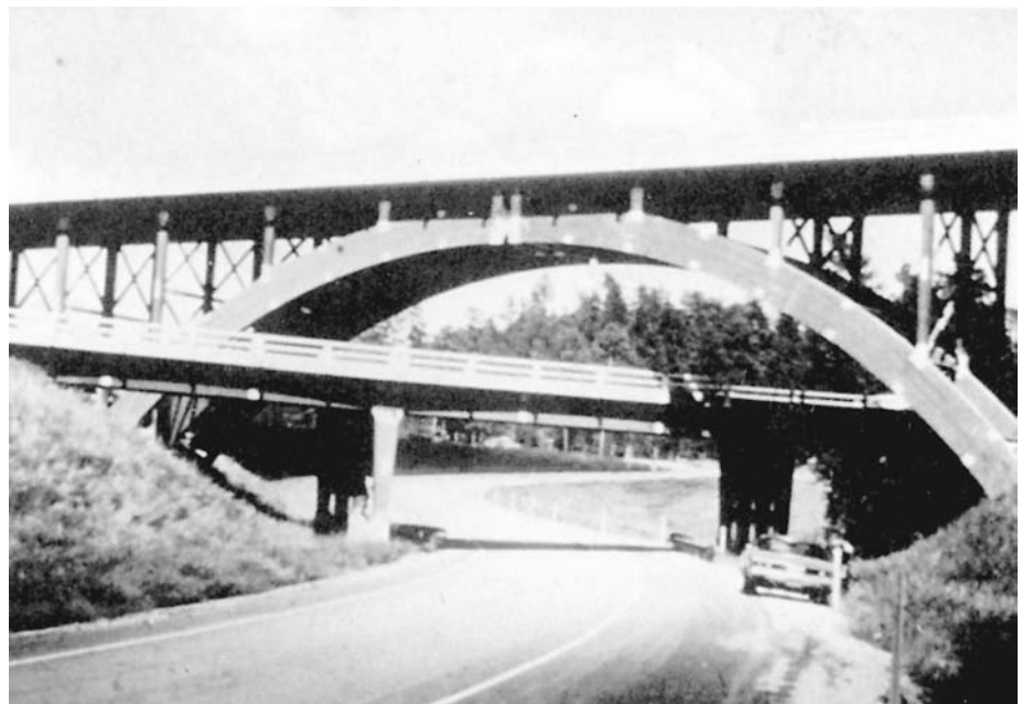
FIGURE 31. Highway bridges supported by glued laminated timber beams. (Courtesy of American Institute of Timber Construction)
