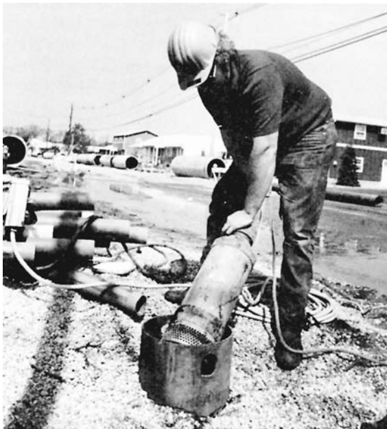
FIGURE 23. Electrically powered submersible pump being placed into dewatering well. (Courtesy of Crane Pumps and Systems)
