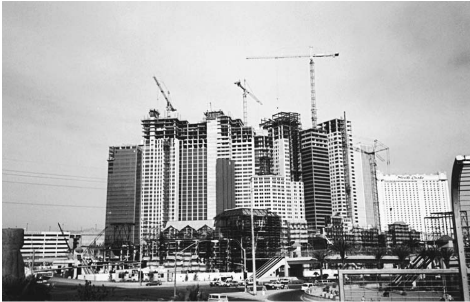
FIGURE 3. Modern building construction project.
