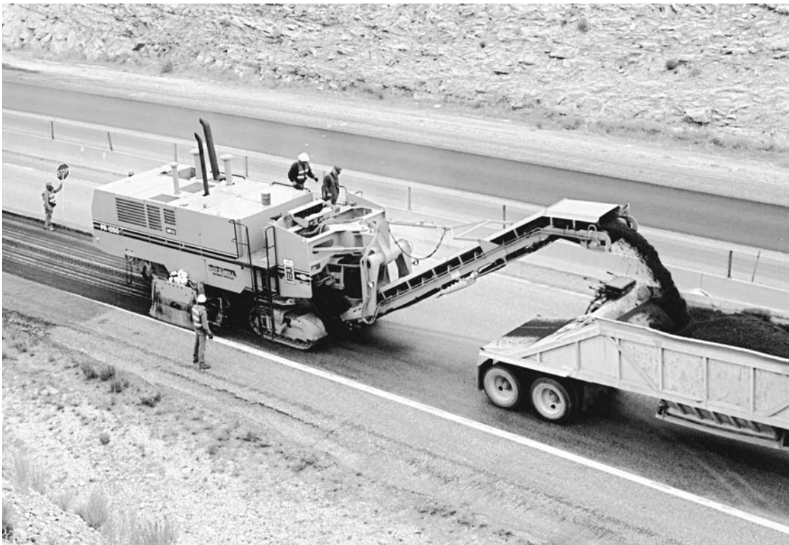
FIGURE 9. Pavement profiler removing old asphalt pavement. (Courtesy of CMI Terex Corporation)
