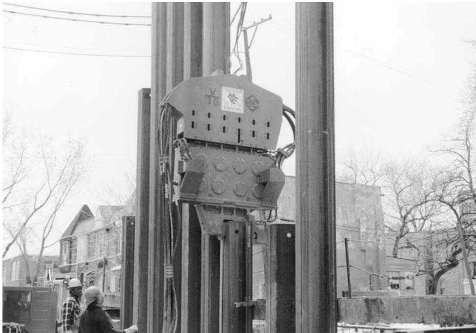
FIGURE 7. Hydraulically powered vibratory driver/extractor. (Courtesy of MKT Manufacturing, Inc.)
