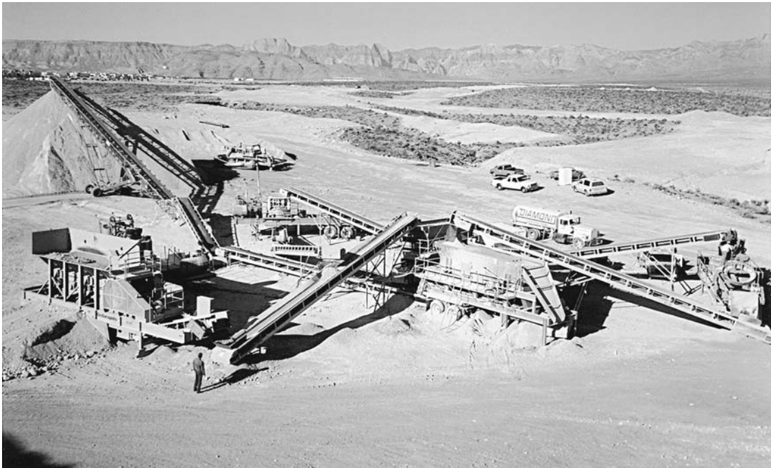
FIGURE 1. Aggregate processing plant. (Courtesy of Cedarapids, Inc.)
