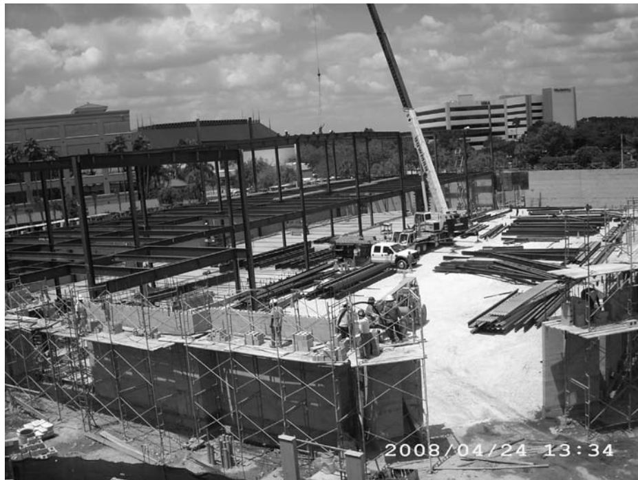
FIGURE 1. Erection of the structural steel frame for a shopping center.
