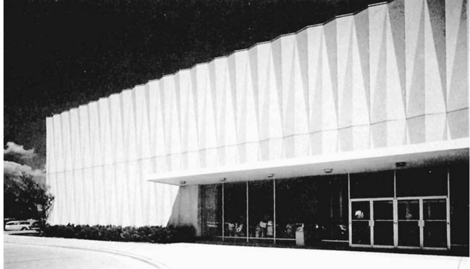
FIGURE 12. Application of architectural concrete. (Courtesy of Portland Cement Association)
