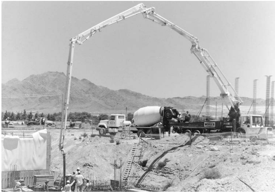
FIGURE 15. Concrete pump and truck mixer. (Courtesy of Morgen Manufacturing Co.)
