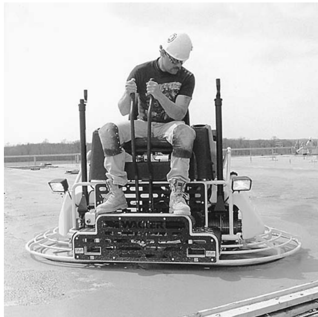
FIGURE 16. Ride-on power trowel. (Courtesy of Wacker Corporation)
