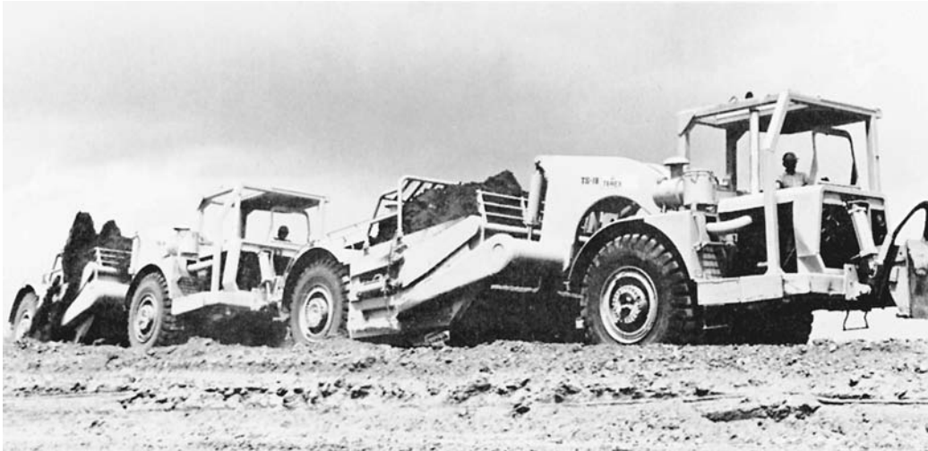
FIGURE 20. Twin-hitch scraper loading. (Courtesy of CMI Terex Corporation)
