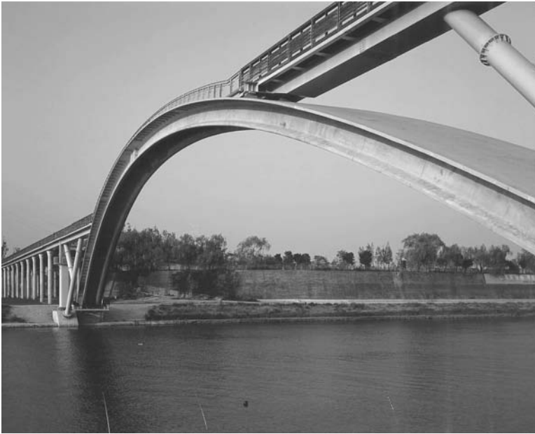
Figure 12-21 Application of ultra-high-performance fiber-reinforced composite to a slender bridge.
