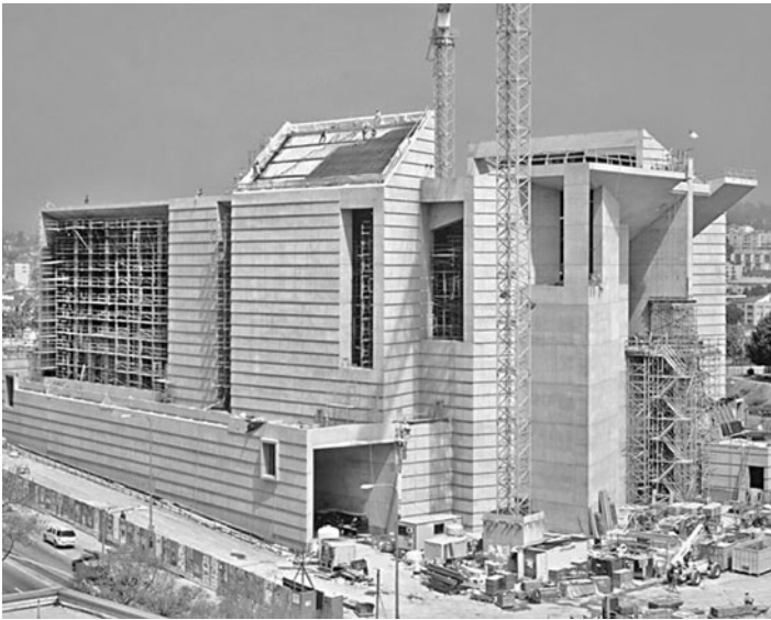
Figure 13-21 Use of architectural mass concrete in the Los Angeles Cathedral. (From Selna, D., and P.J.M. Monteiro, Cathedral of Our Lady of The Angels, Concr. Int. , November, 2001.)
