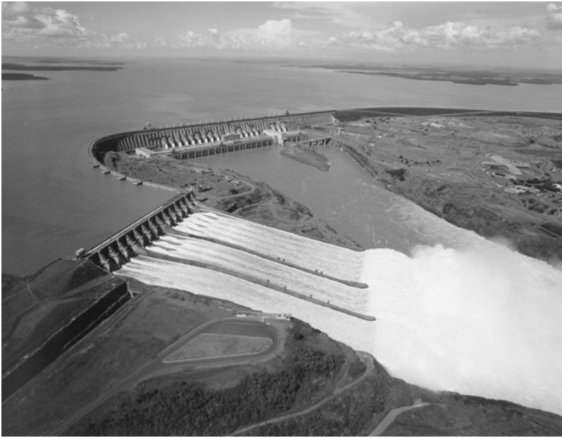
Figure 1-1 Itaipu Dam, Brazil. (Photograph courtesy of Itaipu Binacional, Brazil.)
