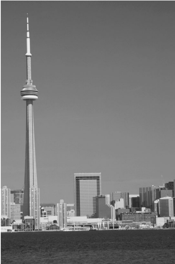
Figure 10-13 The CN Communication Tower, Toronto, Canada, 1974. (Photograph from Hemera Technologies)
