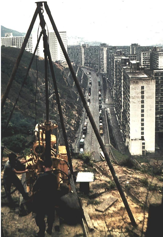
Figure 11: Drilling vertical diamond core holes into the Sau Mau Ping slope. These holes were used for geotechnical investigation purposes and also for the installation of piezometers in the rock mass.
