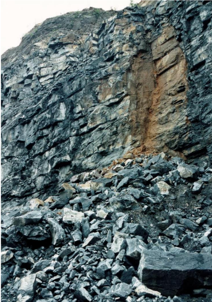
Figure 31: Structurally controlled failure in the face of a steep bench in a heavily jointed rock mass.
