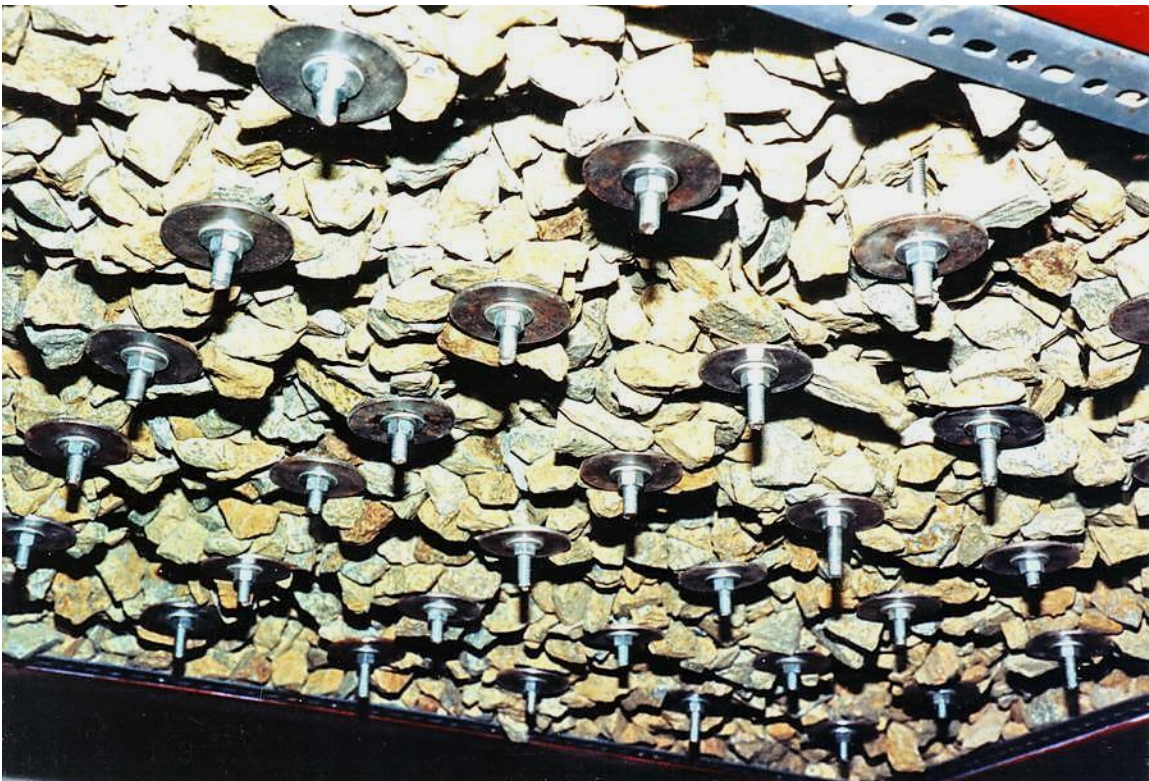
Figure 13: The temporary base removed from the self-supporting rock plate.
