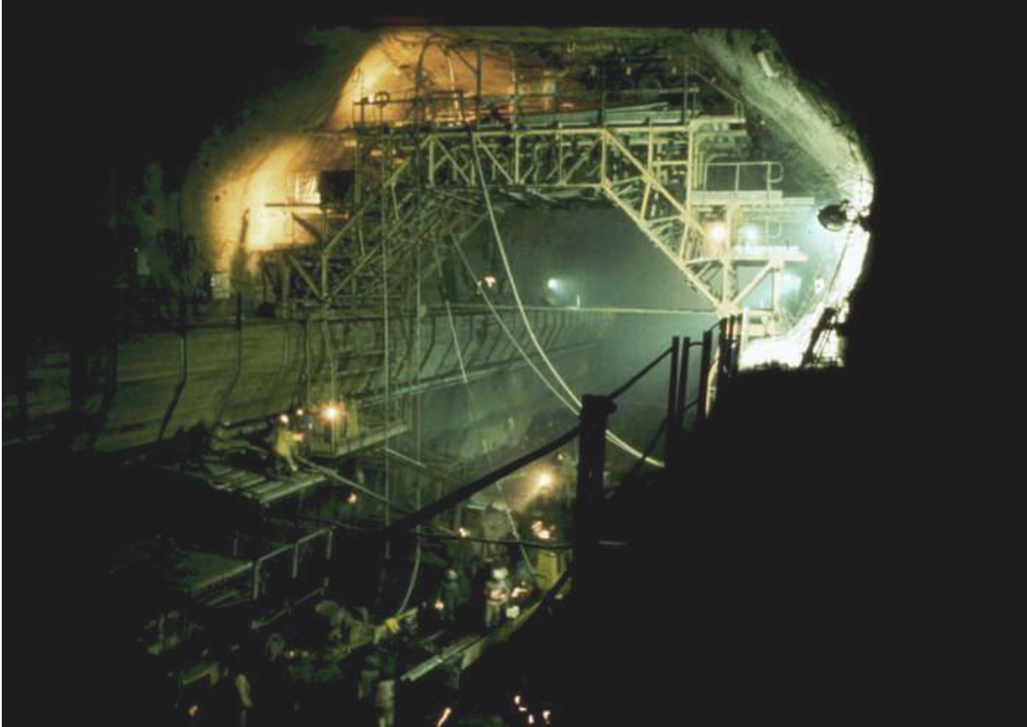
Figure 27: Temporary construction crane running on the main crane beams of the Drakensberg power cavern.
