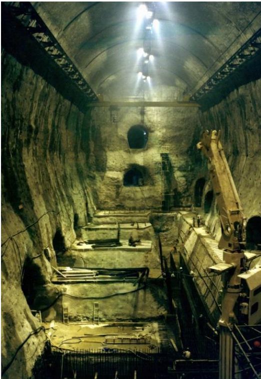
Figure 27: Temporary construction crane running on the main crane beams of the Drakensberg power cavern.
