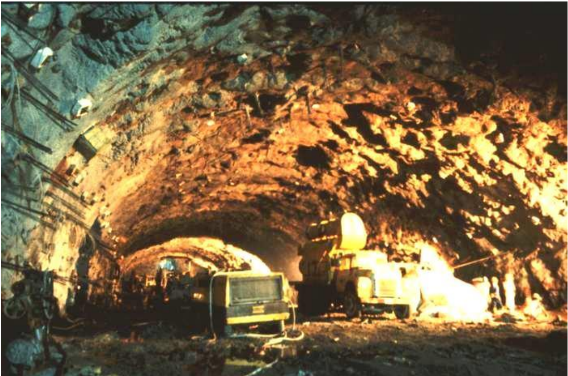
Figure 19: Completed excavation of the cavern arch.
