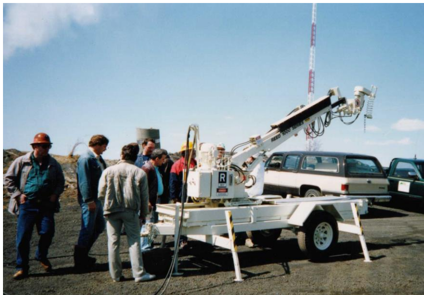
Figure 10: Compact trailer-mounted robot unit for remote controlled shotcrete application.
