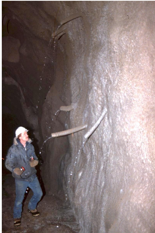
Figure 12: Plastic pipes used to provide drainage for a shotcrete layer applied to a rock mass with water-bearing joints.
